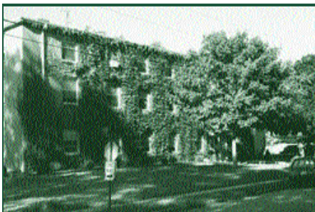
The Chapter House still stands proud after more than 30 years. Recent repairs will ensure its lasting for years to come
